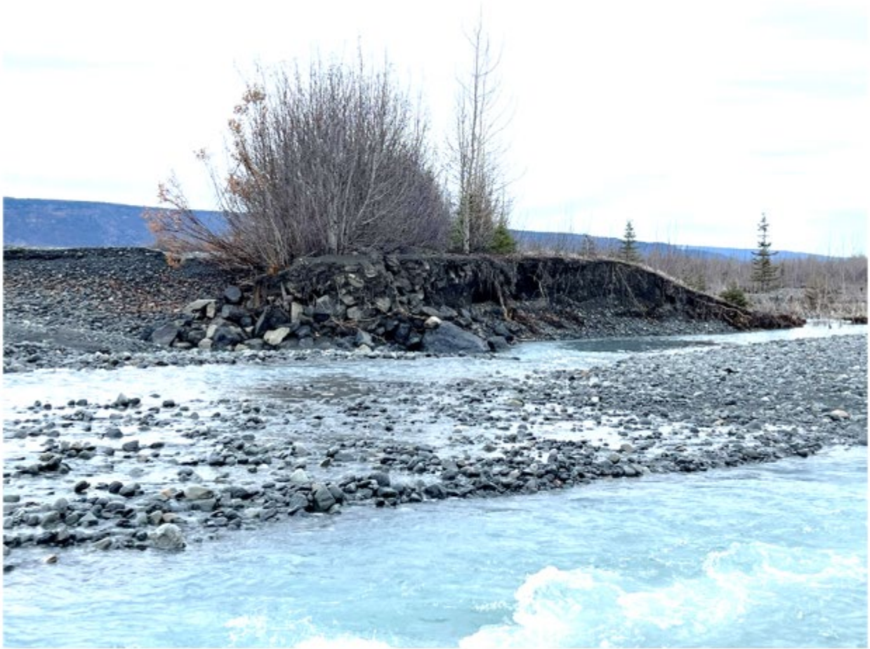
Photo 5-2 Cross-section of levee at breach location, November 2, 2023.
